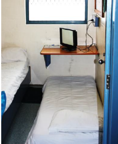
Figure 2: A doubled-up single residential cell at BWCC, taken during the Queensland Ombudsman's 2013 investigation. At the time of their 2015 investigations there had been no changes to the fixtures since that time. 55
